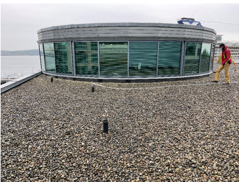
WTCW Roof Photos of Existing Gravel Ballast and Membrane
