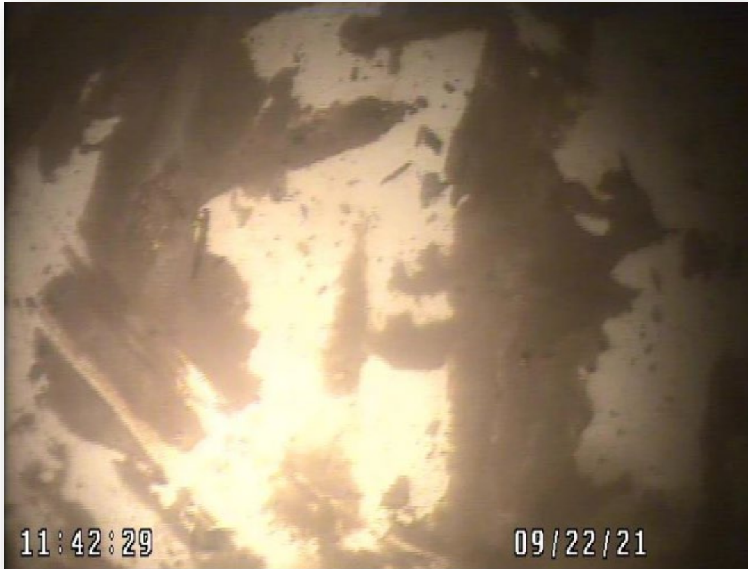
Significant rust on interior tank surfaces
