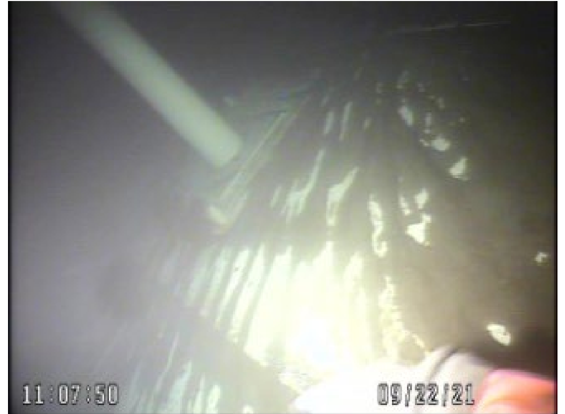
Significant rust on interior tank surfaces
