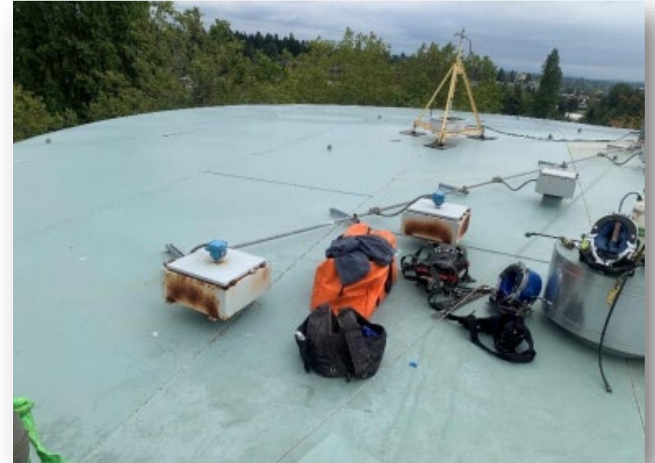
Telemetry boxes Deteriorated coating
