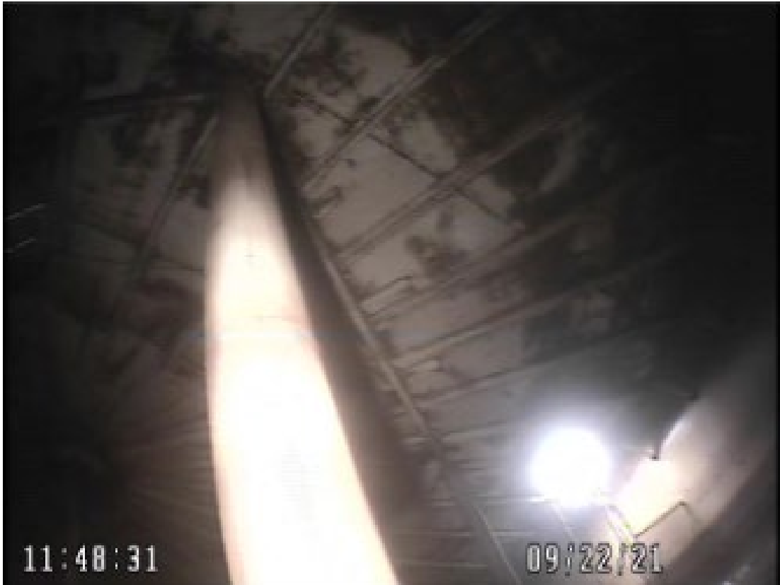
Significant rust on interior tank surfaces
